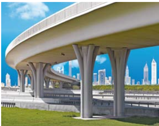
Ras Al Khor bridge, Dubai
