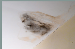
Tanda Air/ Kebocoran
