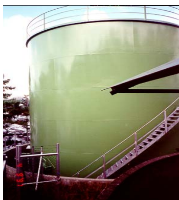
Picture 5: Crude oil storage tank, west coast of Norway, painted in 1995 with a hybrid paint system and with a water-borne styrene acrylic topcoat. The coating system is in excellent condition after 8 years service and the topcoat has maintained its colour and gloss.
