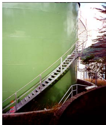
Picture 5: Crude oil storage tank, west coast of Norway, painted in 1995 with a hybrid paint system and with a water-borne styrene acrylic topcoat. The coating system is in excellent condition after 8 years service and the topcoat has maintained its colour and gloss.
