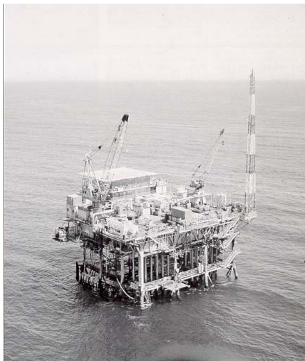
Picture 1: Offshore oil platform in the Bass Strait between South-Australia and Tasmania painted with a water-borne high-build high-ratio IOZ silicate primer in 1990
